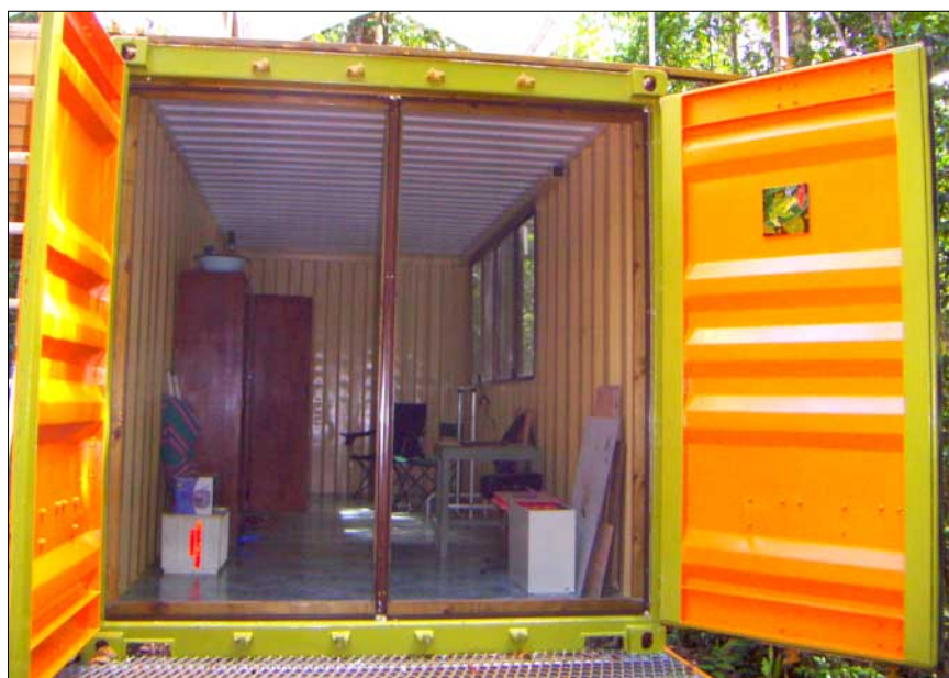
Acrylic roofing paint was used to paint the container in light colours. The acrylic paint has a better ability to expand and contract with the metal.
